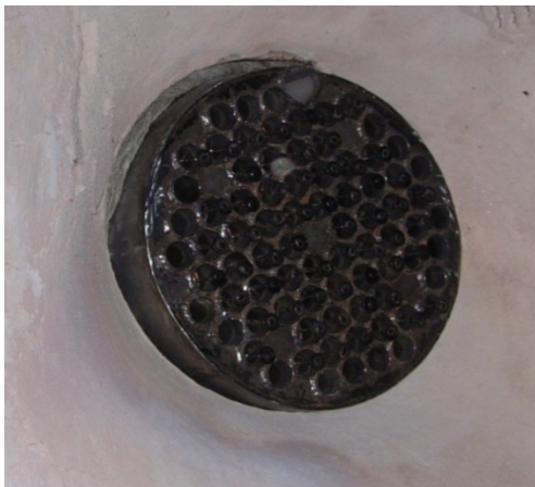
Fig. 2 – View of the MTC burner in a boiler with a capacity of 10 MW and the nature of its flame
