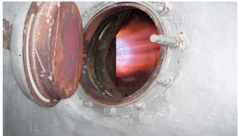
Fig. 2 – View of the MTC burner in a boiler with a capacity of 10 MW and the nature of its flame
